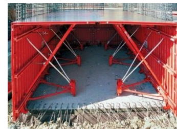
Figure 3: Tunnel formwork system
