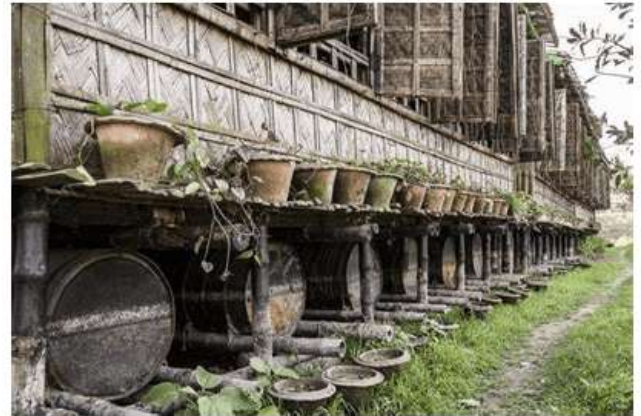
Figure 8: Use of recycled oil drums to elevate the school during flooding
