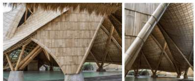
Figure 12: Hybrid bamboo-steel structure of The ARC
