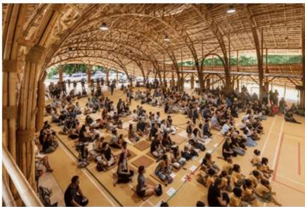
Figure 18: Spacious, columns free, cross ventilated space encourages community activity at Sports Hall
