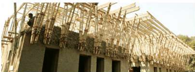
Figure 3: Main structural material-bamboo with earth & straw
