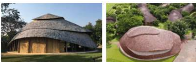
Figure 15: View of Bamboo Sports hall, Chiang Mai
