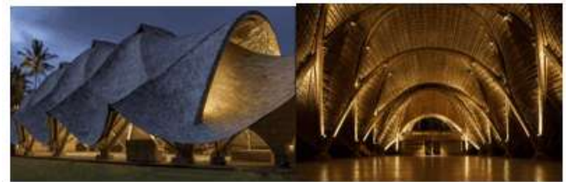
Figure 11: Striking parabolic arches of ARC
