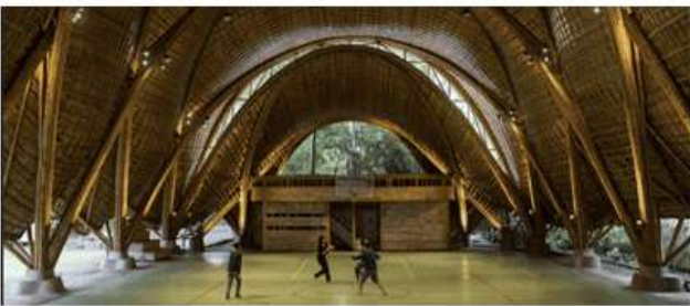
Figure 14: A column-free space promoting activities of the community at ARC
