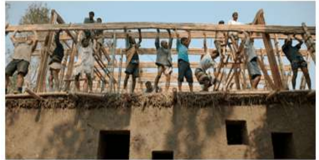
Figure 4: Local artisans constructing the school, METI
